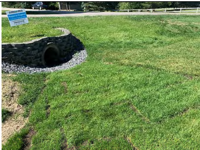
29 Gundalow -1 (Drainage Area)
