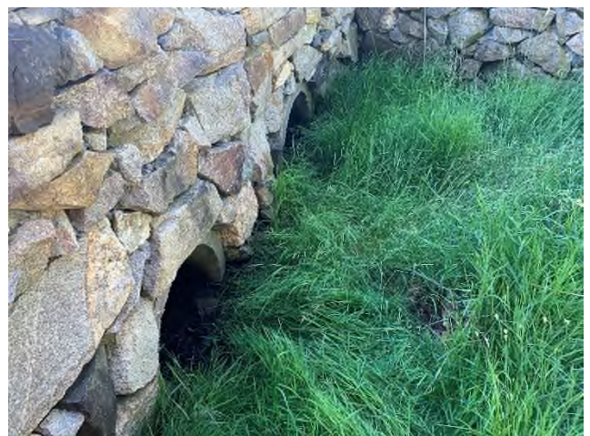
4 Brickyard Circle - 1 (Drainage Course)
