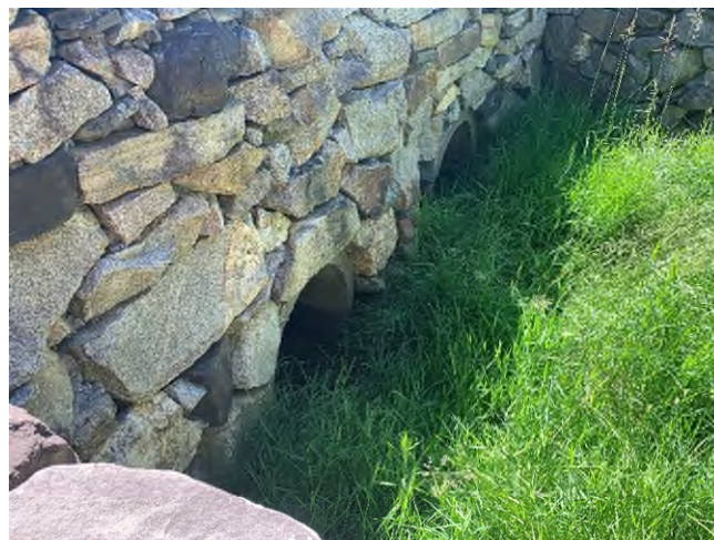
4 Brickyard Circle - 1 (Drainage Course)
