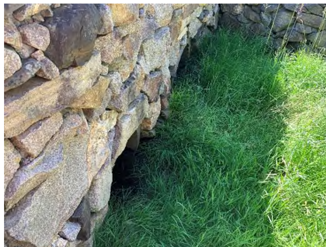
4 Brickyard Circle - 1 (Drainage Course)
