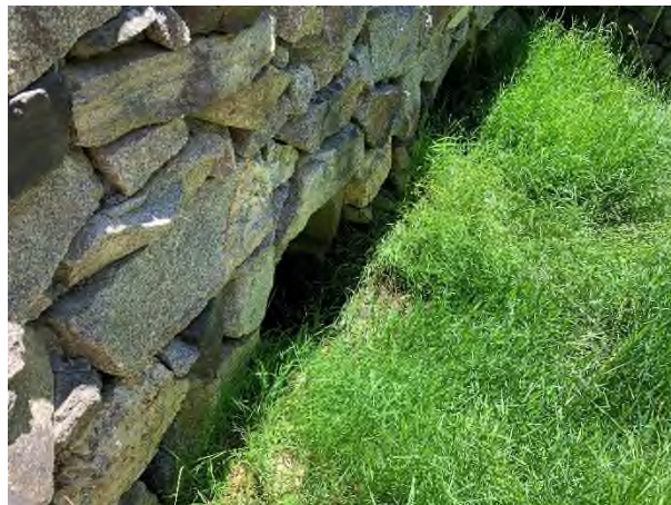
4 Brickyard Circle - 1 (Drainage Course)
