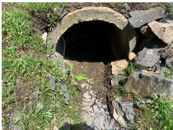
64 Gundalow - 1 (Drainage Course)
