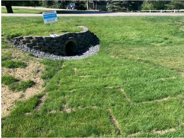
29 Gundalow -1 (Drainage Area)
