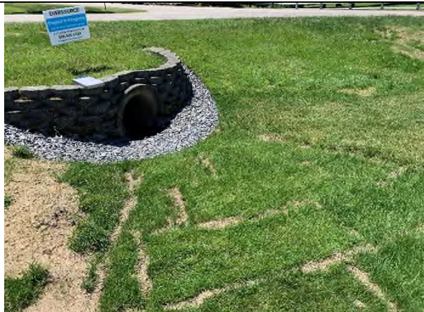
29 Gundalow -1 (Drainage Area)
