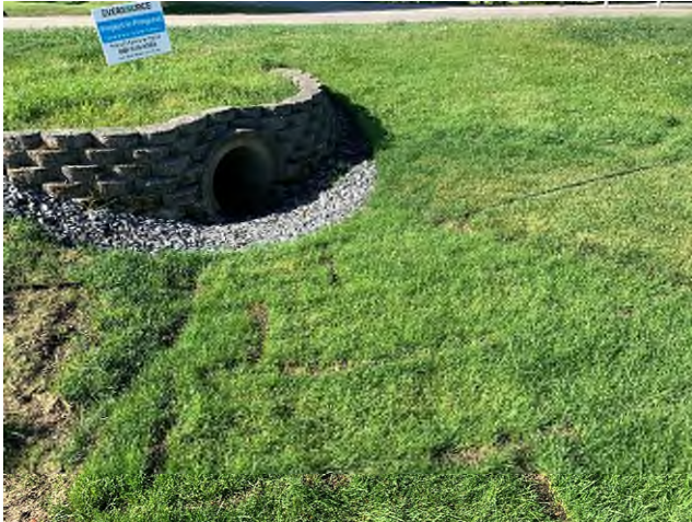
29 Gundalow -1 (Drainage Area)
