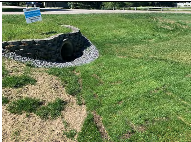
29 Gundalow -1 (Drainage Area)
